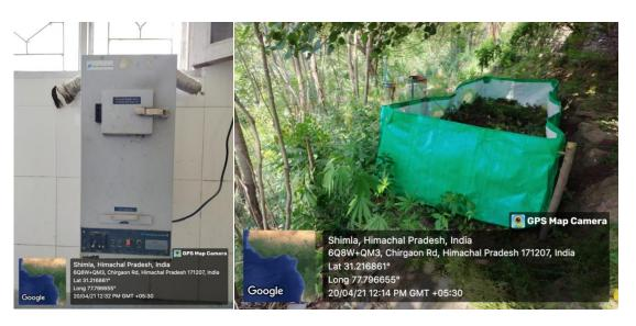
2. <u>Sanitary pad incinerator and vermi-composting unit for management of sanitary pads and Organic waste</u>
