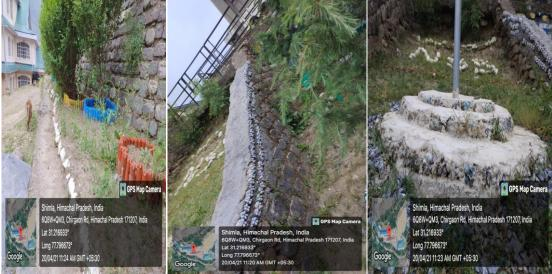
3. Reuse of plastic by NSS volunteers under waste to wealth concept plastic bottles filled with compacted plastic wrappers used as flower/plant beds and in concrete wall and flag pedestal
